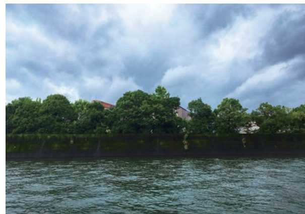
The breakwater, constructed along the contour of Otake Plant, near the estuary of Egawa River and the green belt
