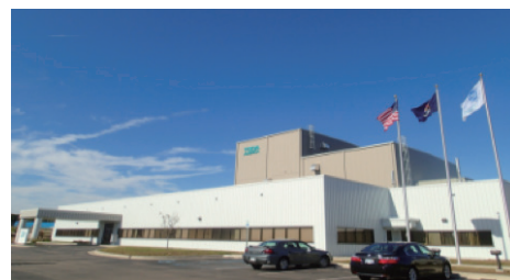
External appearance of BTA
