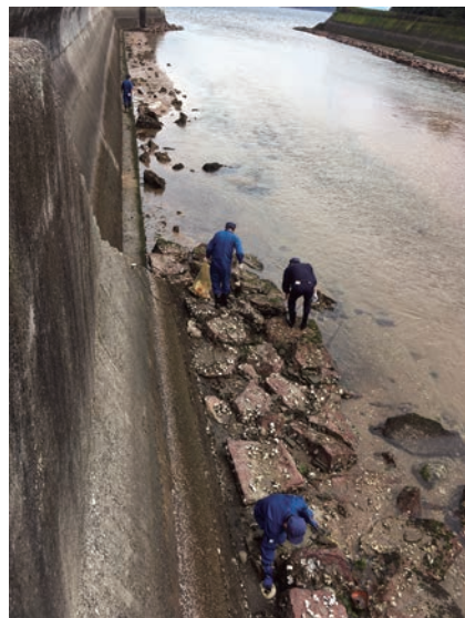
Cleanup activities of Egawa River adjacent to Otake Plant
