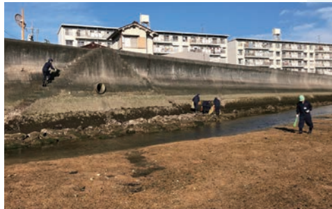
Cleanup activities of Egawa River adjacent to Otake Plant
