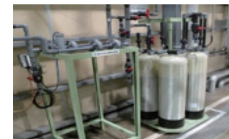
Cartridge unit for adsorbent for water treatment
