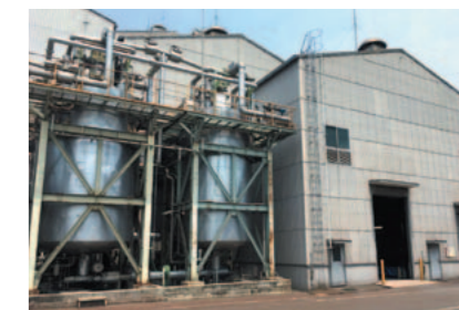
Environmentally functional materials manufacturing plant
