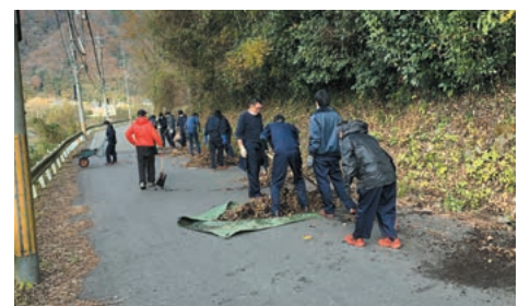
Road gutter cleanup activities
